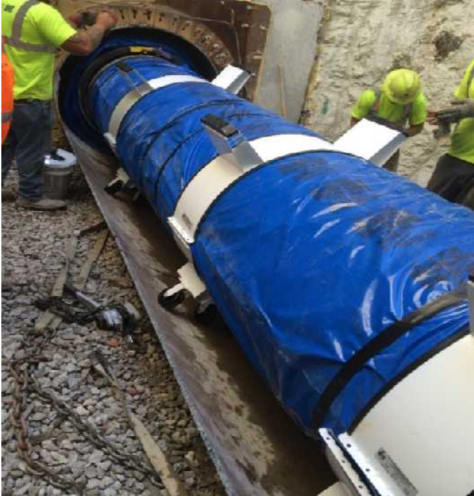
1,500 foot river crossing
